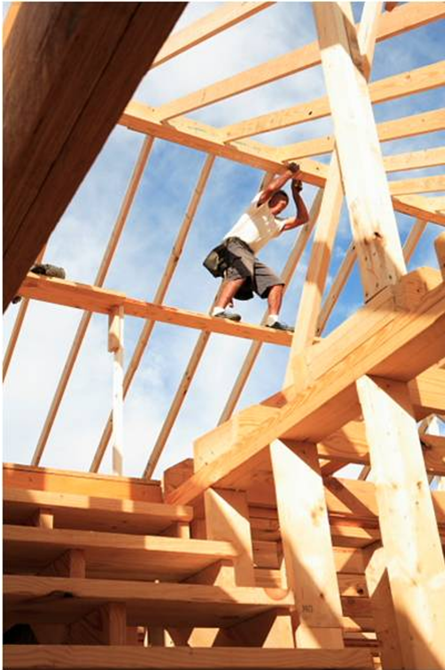
Image 868: OSHA Training Institute, Southwest Education Center http://www.elcosh.org
